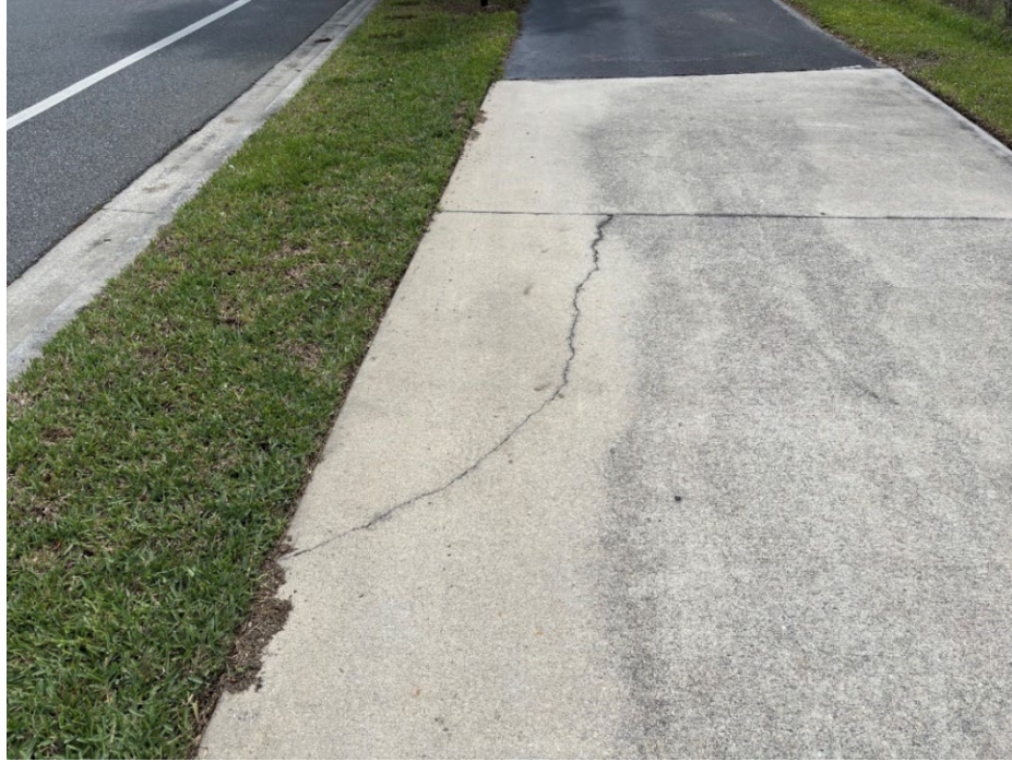
Photo 53 - Cracked Concrete and Base Failure (No Observed Changes) (Refer to Prior Photo 73 – 2025 Assessment)
