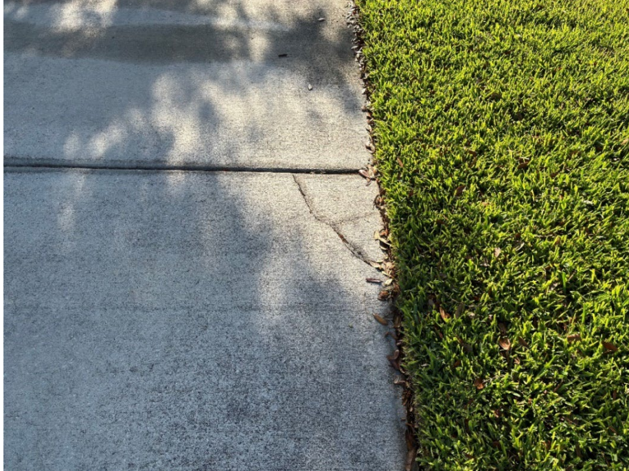
Photo 14 - Cracked Concrete and Base Failure (No Observed Changes) (Refer to Prior Photo 18 – 2025 Assessment)
