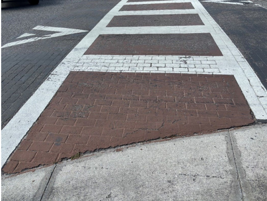
Photo 37 Deteriorating Thermoplastic and Worn Crosswalk Coloration (No Observed Changes) (Refer to Prior Photo 52 – 2025 Assessment)
