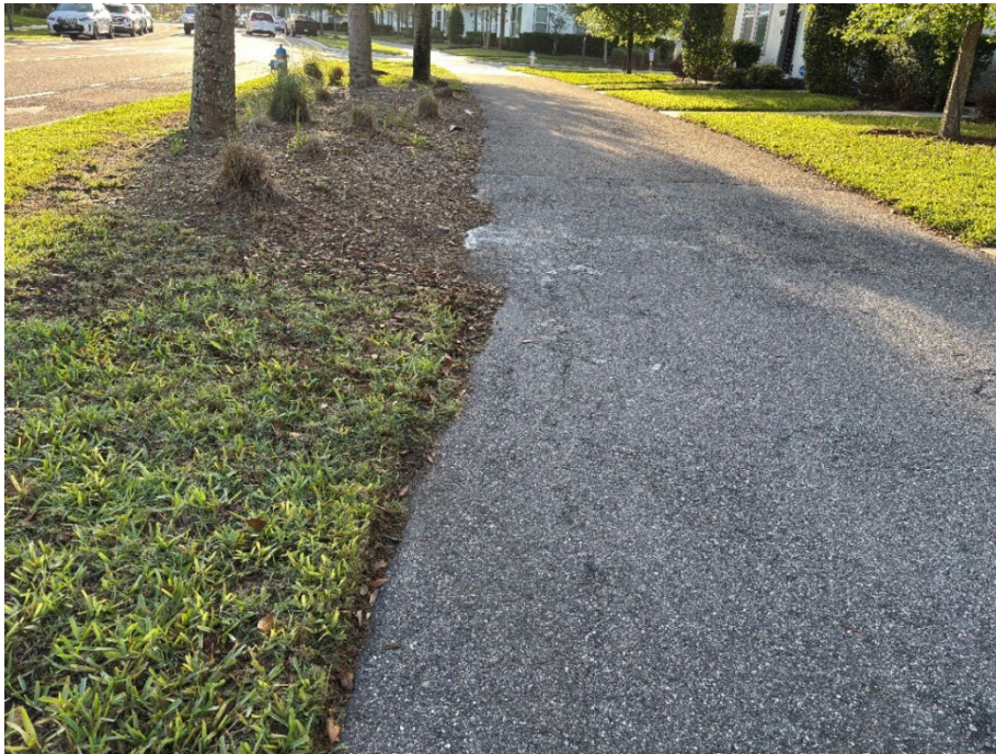
Photo 5 - Asphalt Pavement Edge Failure (No Observed Changes) (Refer to Prior Photo 5 – 2025 Assessment)
