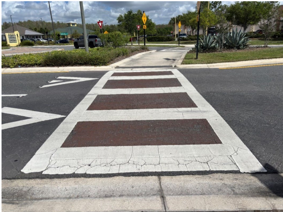
Photo 54 Deteriorating Thermoplastic and Worn Crosswalk Coloration (No Observed Changes) (Refer to Prior Photo 74 – 2025 Assessment)
