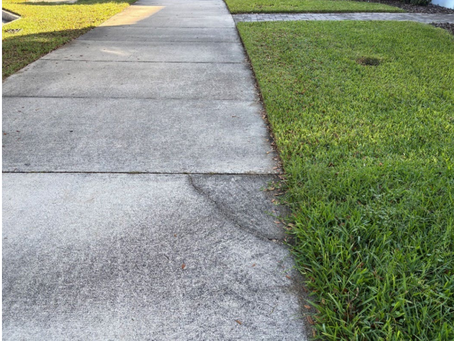
Photo 12 Cracked Concrete and Base Failure (No Observed Changes) (Refer to Prior Photo 16 – 2025 Assessment)
