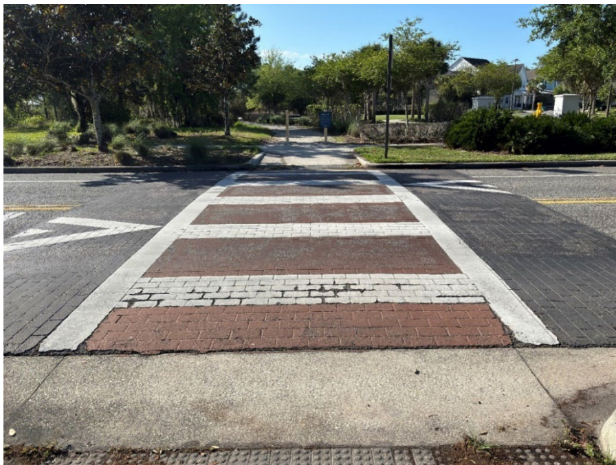
Photo 22 - Deteriorating Thermoplastic and Worn Crosswalk Coloration (Further Deterioration Observed) (Refer to Prior Photo 30 – 2025 Assessment)
