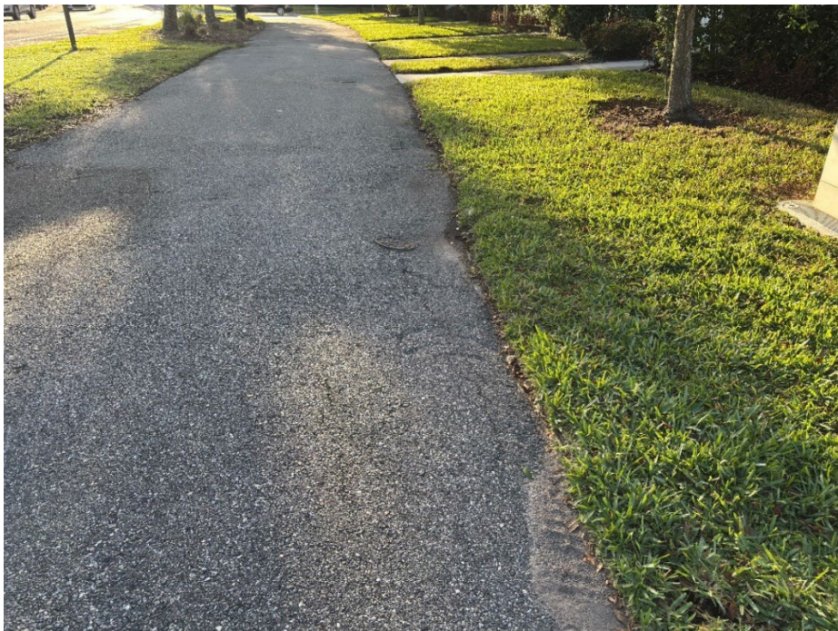
Photo 2 Asphalt Pavement Edge Failure (Increasing Edge Failure Observed) (Refer to Prior Photo 2 – 2025 Assessment)
