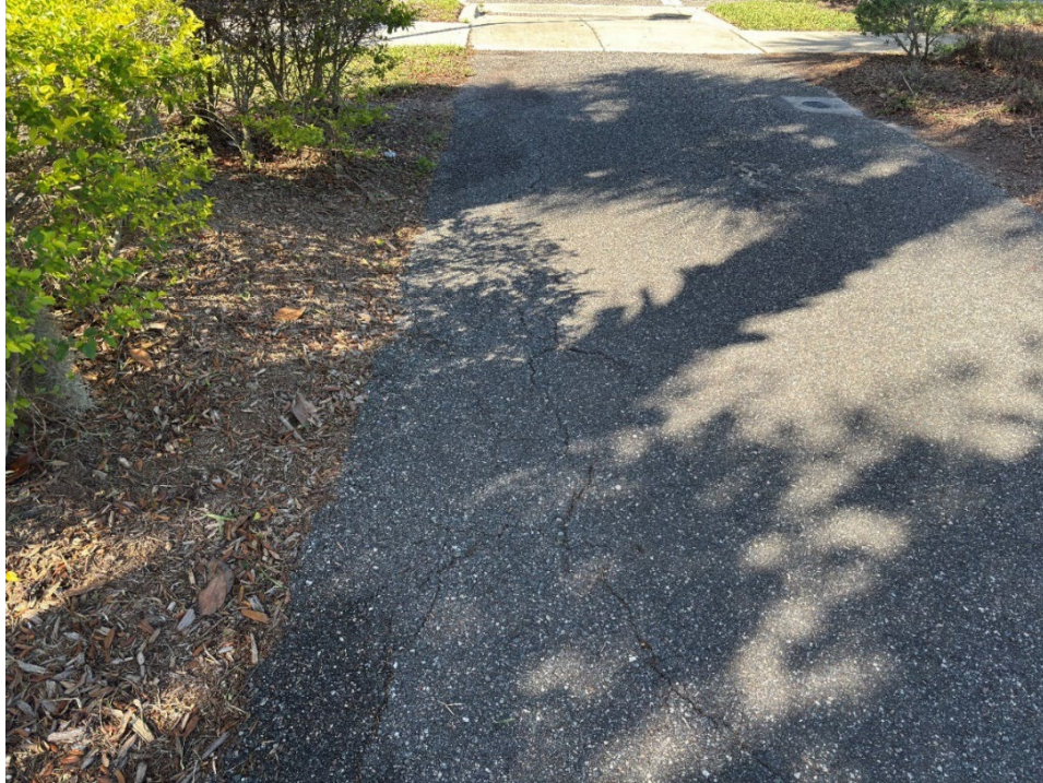
Photo 25 - Asphalt Raveling (No Observed Changes) (Refer to Prior Photo 34 – 2025 Assessment)
