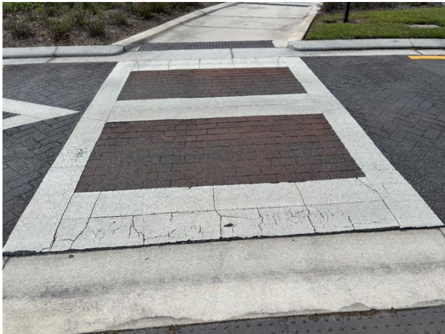
Photo 56 Deteriorating Thermoplastic and Worn Crosswalk Coloration (Further Deterioration Observed) (Refer to Prior Photo 76 – 2025 Assessment)
