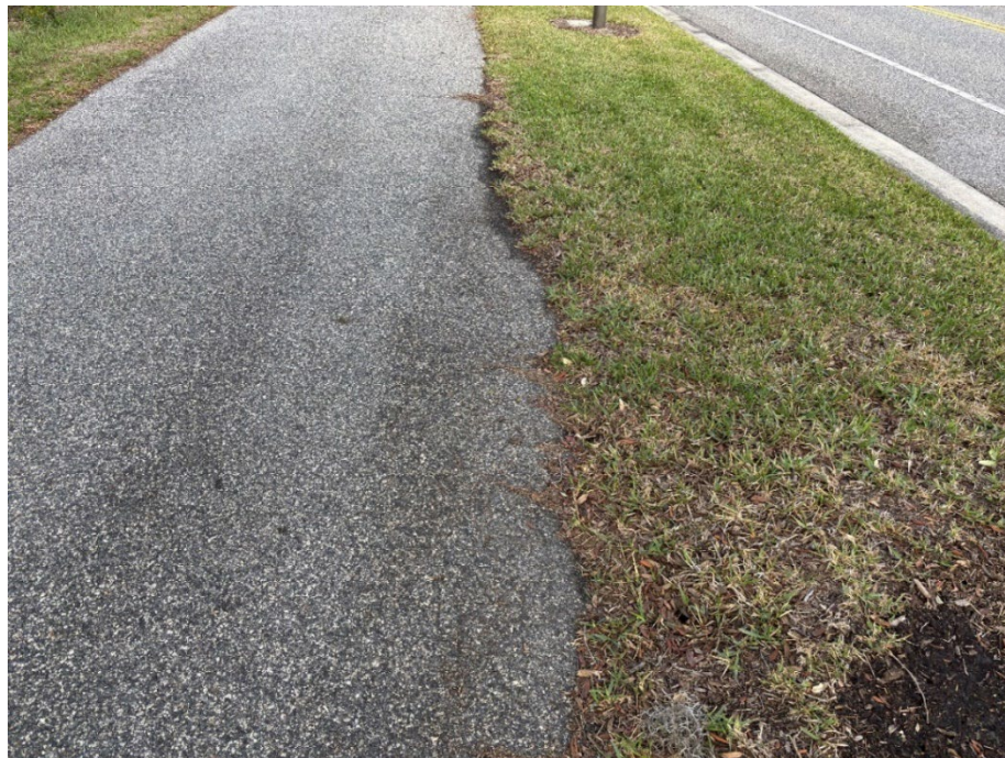
Photo 45 Asphalt Pavement Edge Failure (No Observed Changes) (Refer to Prior Photo 60 – 2025 Assessment)
