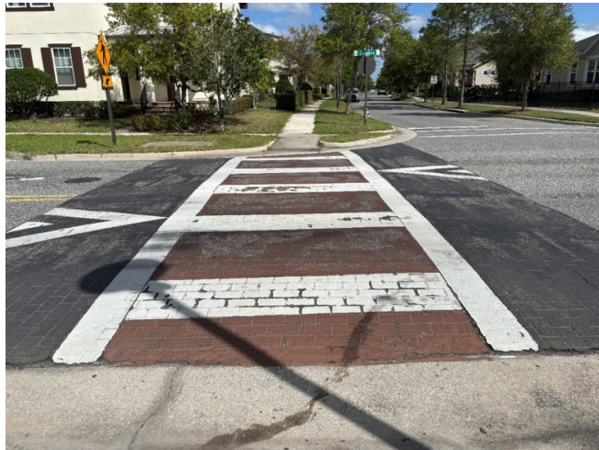
Photo 40 Deteriorating Thermoplastic and Worn Crosswalk Coloration (Further Deterioration Observed) (Refer to Prior Photo 55 – 2025 Assessment)
