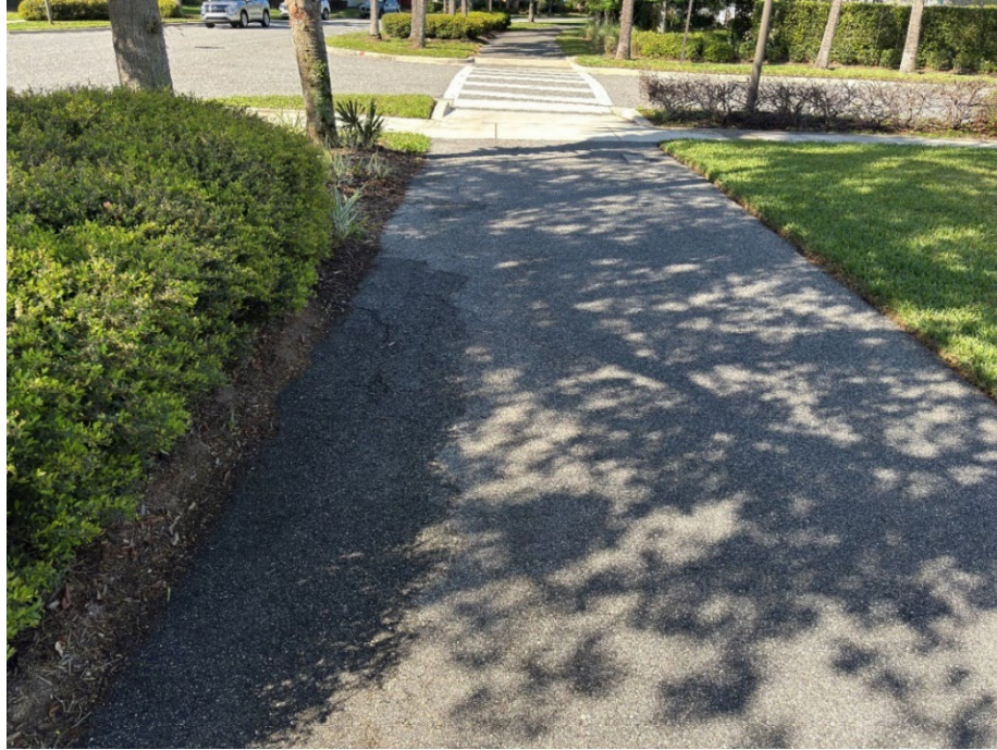
Photo 31 - Asphalt Raveling (No Observed Changes) (Refer to Prior Photo 40 – 2025 Assessment)
