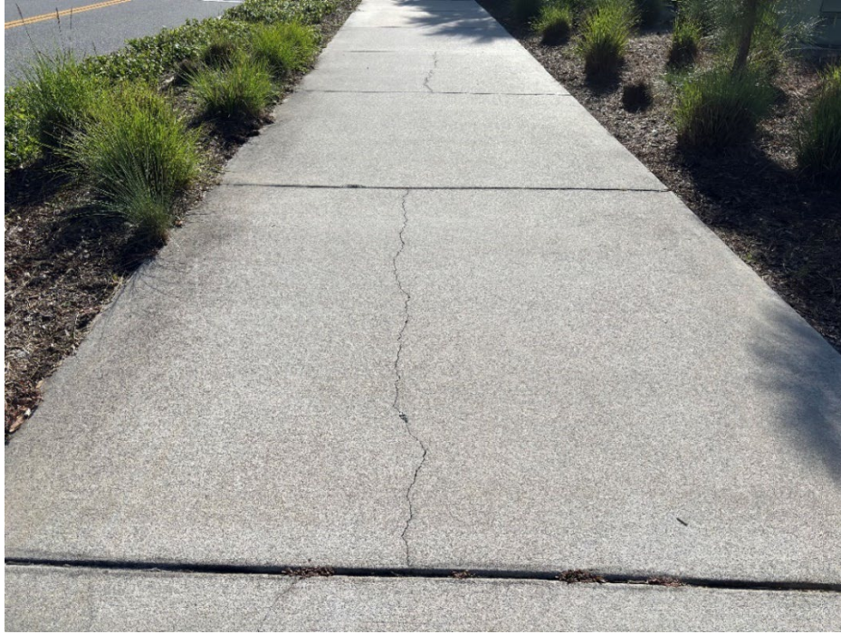
Photo 18 - Surficial Cracked Concrete (No Observed Changes) (Refer to Prior Photo 23 – 2025 Assessment)
