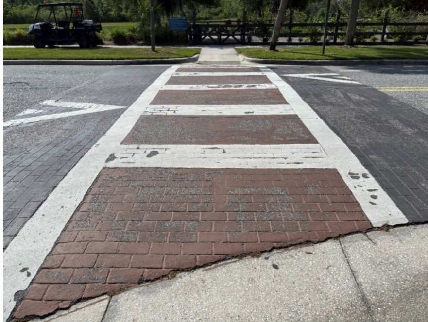
Photo 41 Deteriorating Thermoplastic and Worn Crosswalk Coloration (Further Deterioration Observed) (Refer to Prior Photo 56 – 2025 Assessment)
