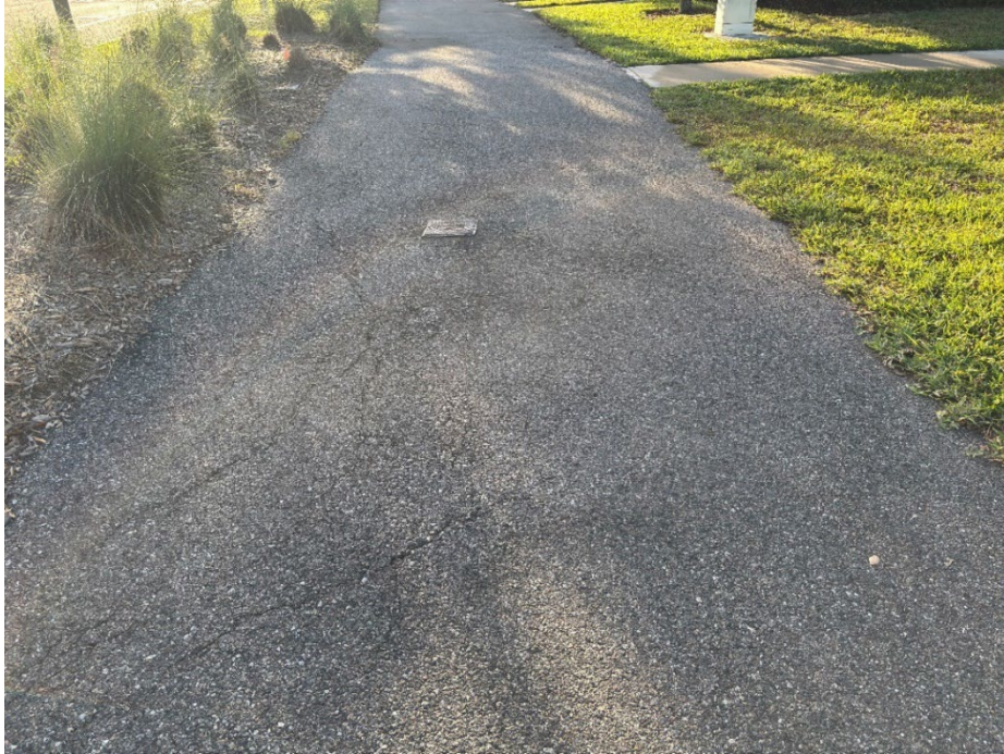
Photo 1 Asphalt Raveling (No Observed Changes) (Refer to Prior Photo 1 – 2025 Assessment)
