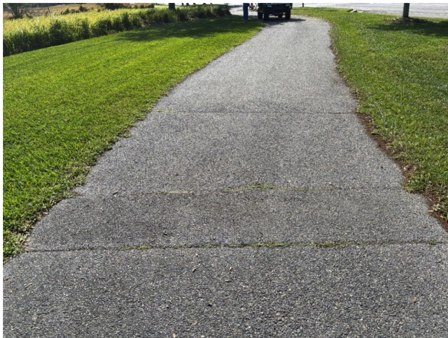
Photo 34 - Cracked Asphalt and Asphalt Raveling (No Observed Changes) (Refer to Prior Photo 47 – 2025 Assessment)
