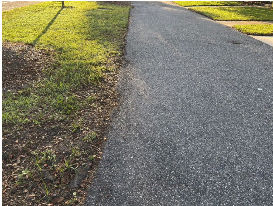
Photo 4 Asphalt Pavement Edge Failure (Increasing Edge Failure Observed) (Refer to Prior Photo 4 – 2025 Assessment)
