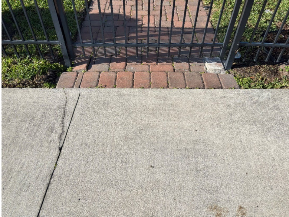
Photo 13 - Surficial Cracked Concrete (No Observed Changes) (Refer to Prior Photo 17 – 2025 Assessment)
