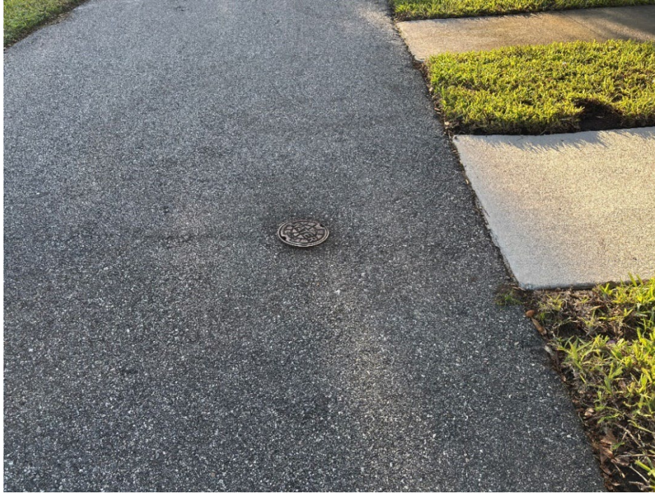
Photo 3 Valve Cover Approximately 1 inch Reveal (No Observed Changes) (Refer to Prior Photo 3 – 2025 Assessment)
