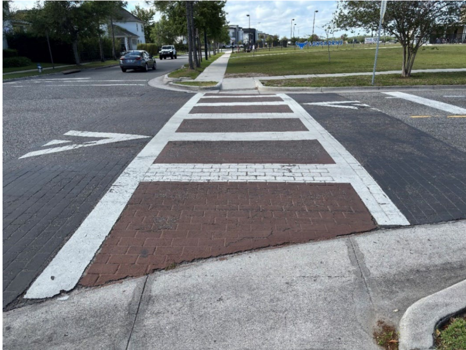
Photo 36 Deteriorating Thermoplastic and Worn Crosswalk Coloration (No Observed Changes) (Refer to Prior Photo 51 – 2025 Assessment)
