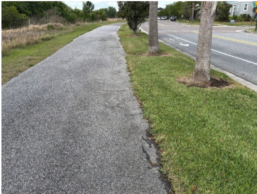
Photo 42 Asphalt Raveling and Base Failure (Further Edge Failure Observed) (Refer to Prior Photo 57 – 2025 Assessment)
