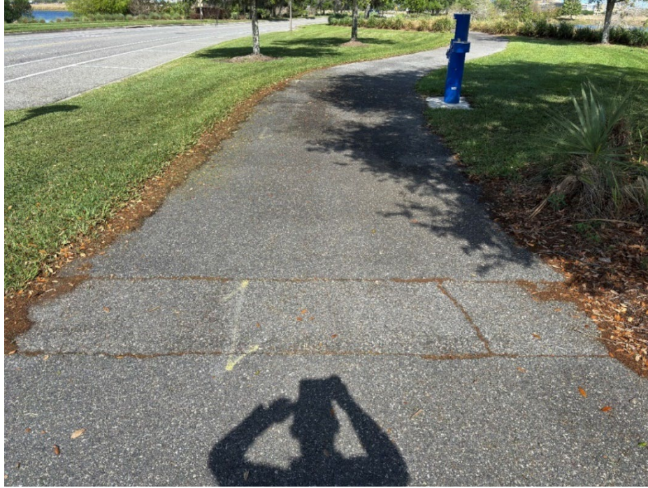
Photo 33.2 - Multiple Cracked Asphalt and Asphalt Raveling (New Photo – 2026 Assessment)
