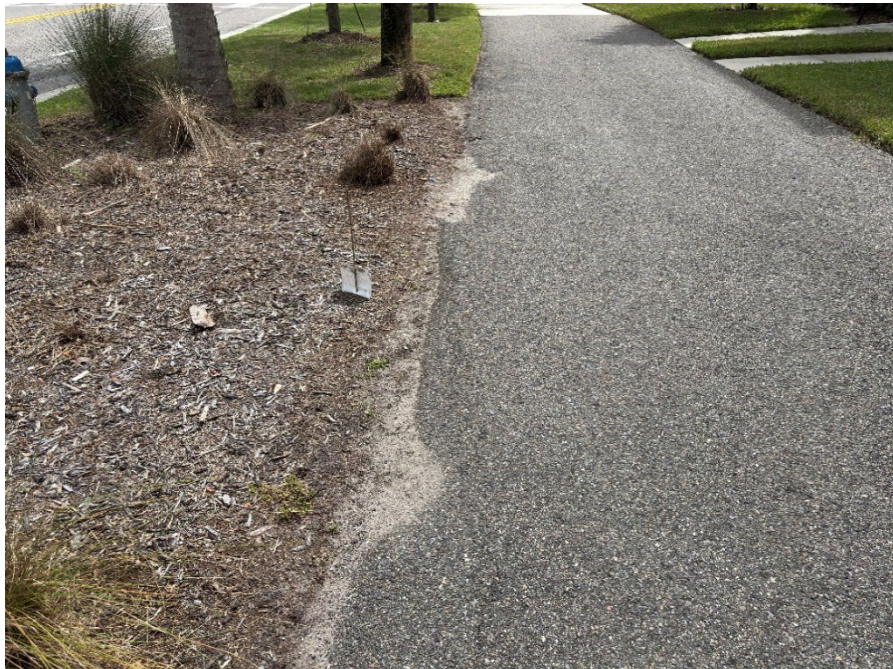
Photo 6 - Asphalt Pavement Edge Failure (No Observed Changes) (Refer to Prior Photo 6 – 2025 Assessment)
