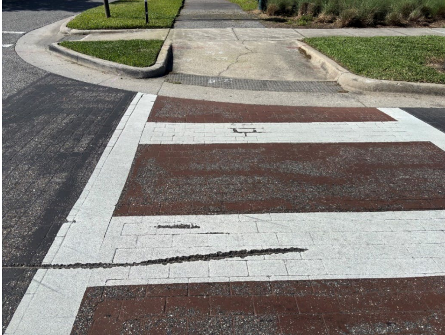
Photo 35 Deteriorating Thermoplastic and Worn Crosswalk Coloration (No Observed Changes) (Refer to Prior Photo 50 – 2025 Assessment)
