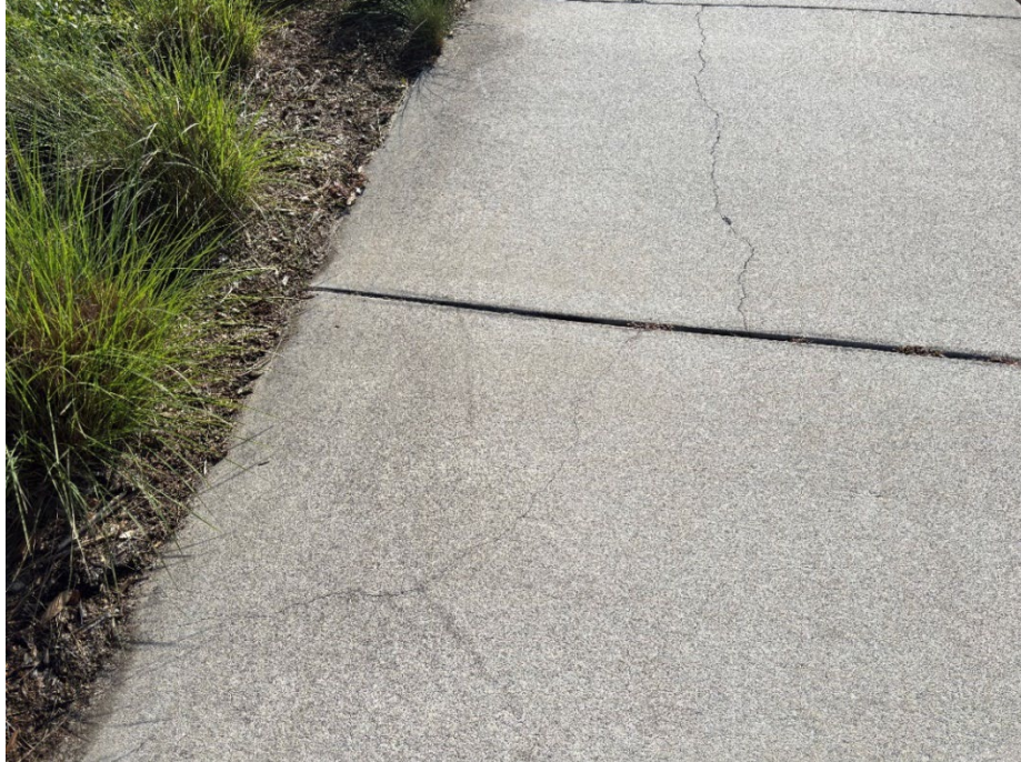
Photo 17 - Surficial Cracked Concrete (No Observed Changes) (Refer to Prior Photo 22 – 2025 Assessment)
