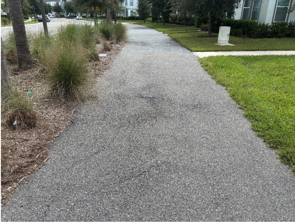
Photo 1 – Asphalt Raveling
