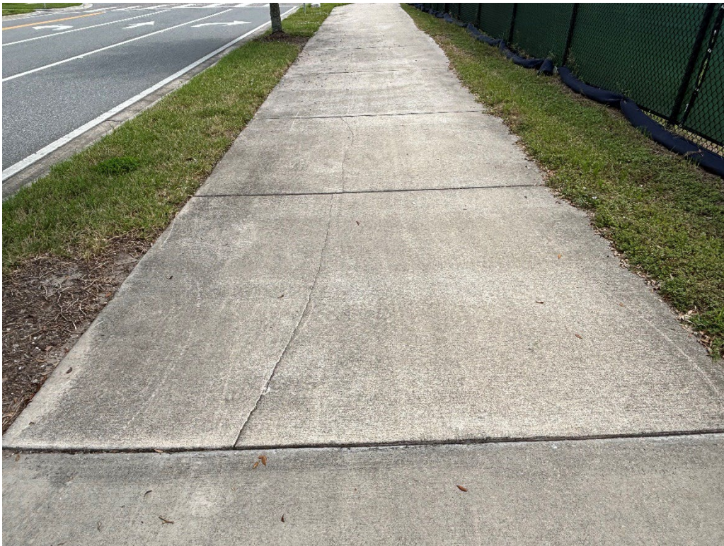
Photo 28 – Cracked Concrete
