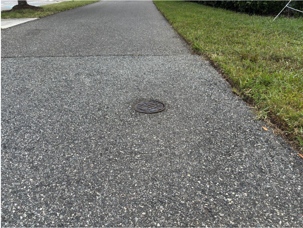
Photo 9 – Valve Cover Approximately 1/2-inch Reveal
