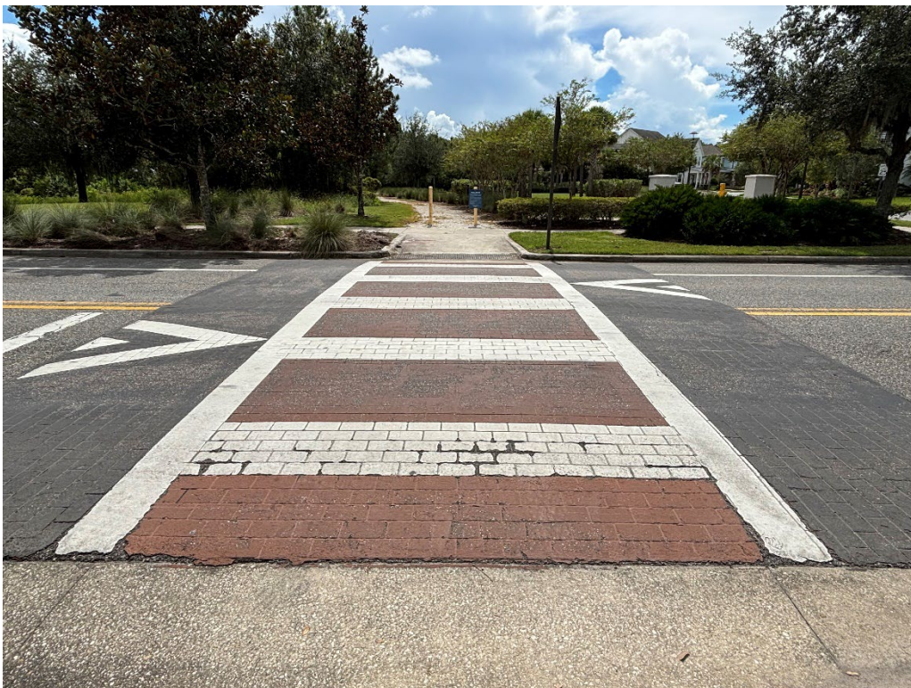
Photo 30 - Deteriorating Thermoplastic and Worn Crosswalk Coloration
