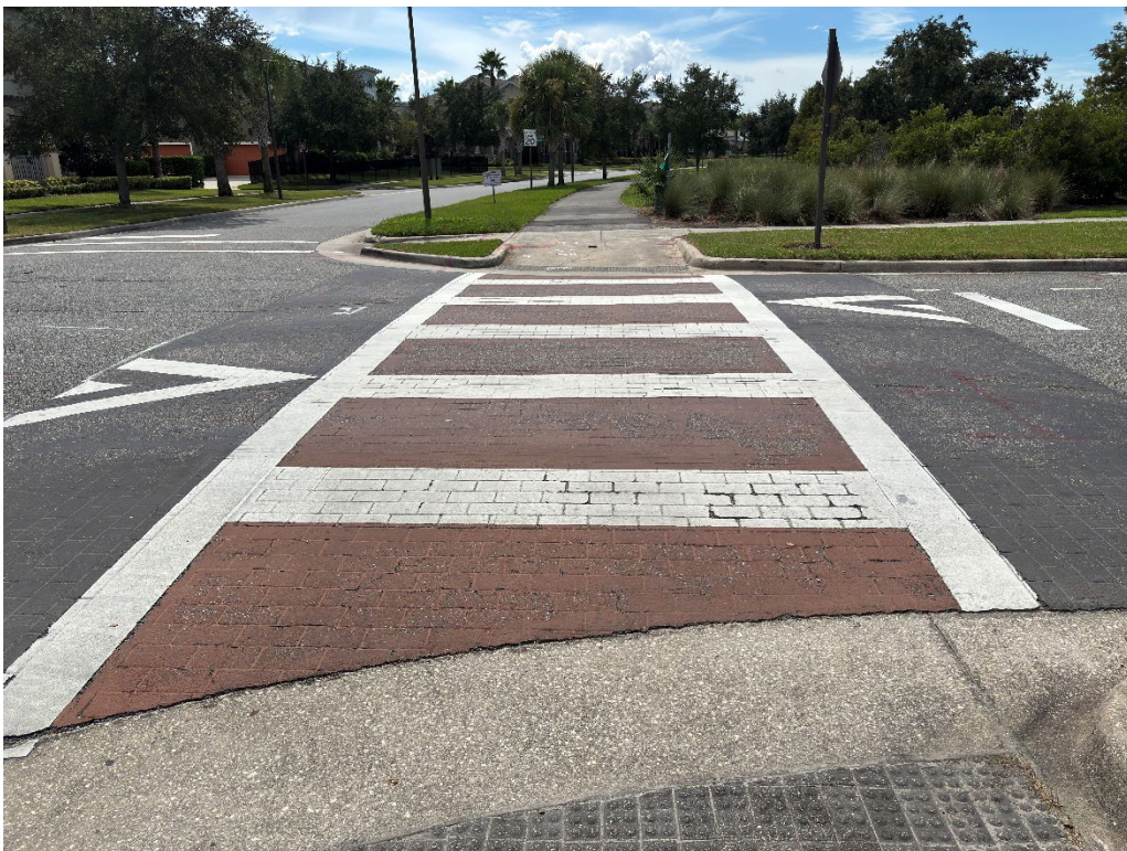
Photo 48 – Deteriorating Thermoplastic and Worn Crosswalk Coloration
