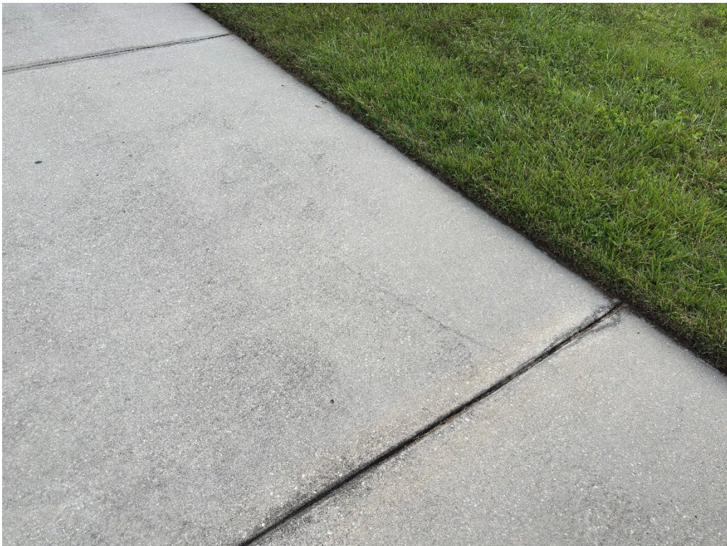
Photo 20 – Surficial Cracked Concrete
