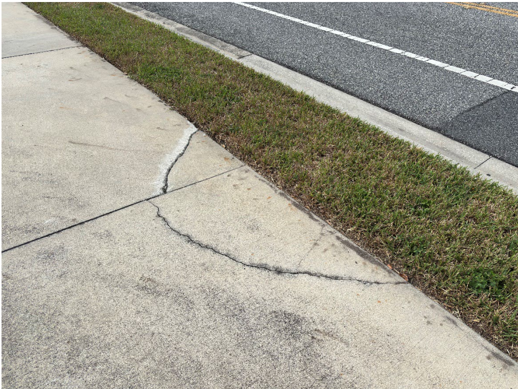
Photo 72 – Cracked Concrete and Base Failure
