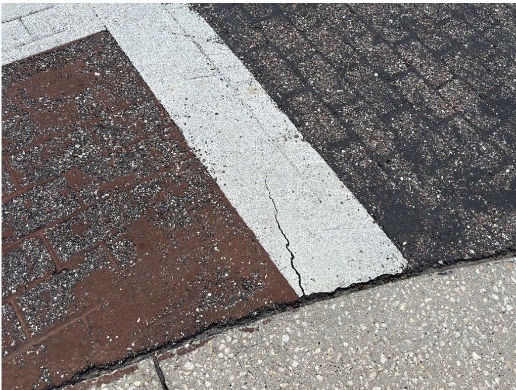
Photo 36 – Deteriorating Thermoplastic and Worn Crosswalk Coloration
