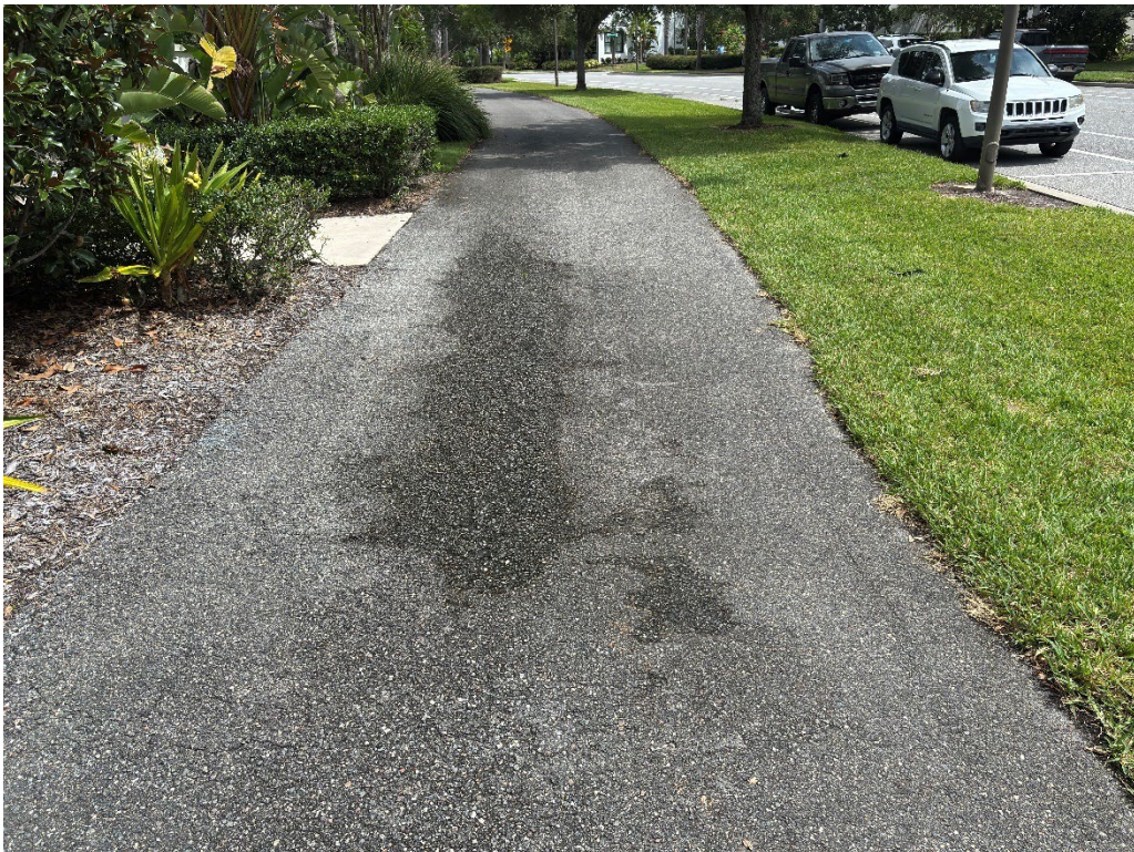
Photo 42 – Asphalt Raveling in Low Area
