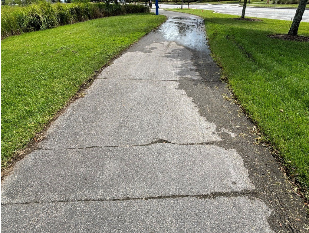
Photo 47 – Cracked Asphalt and Raveling in Low Area
