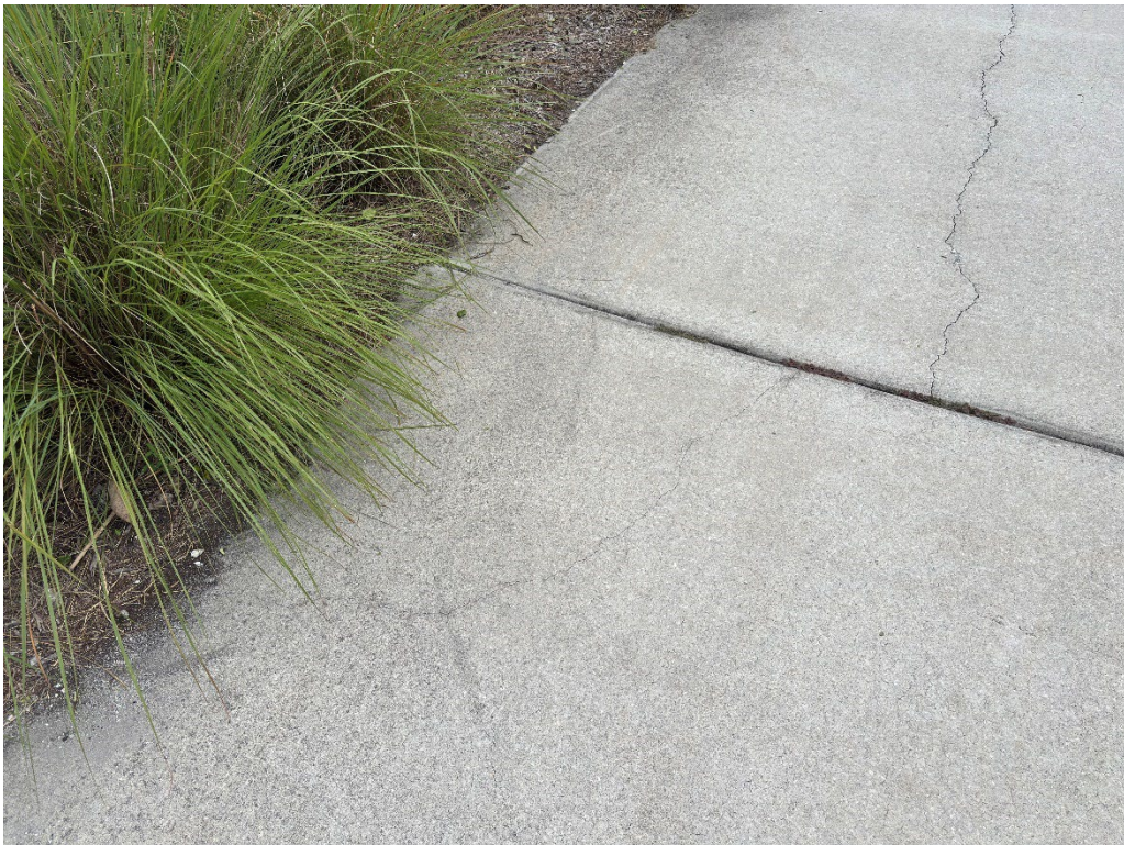
Photo 22 – Surficial Cracked Concrete
