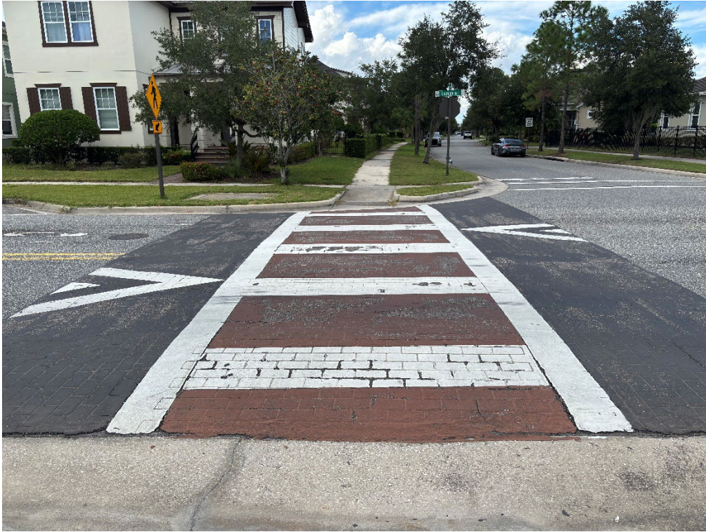
Photo 55 – Deteriorating Thermoplastic and Worn Crosswalk Coloration
