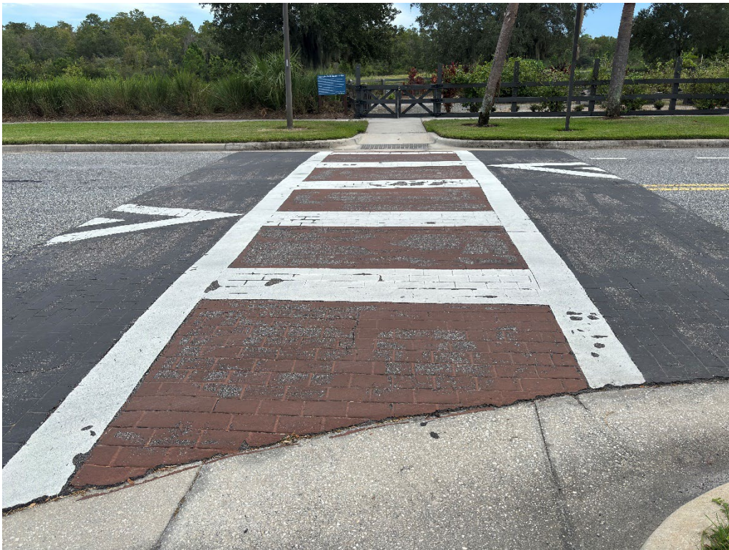
Photo 56 – Deteriorating Thermoplastic and Worn Crosswalk Coloration
