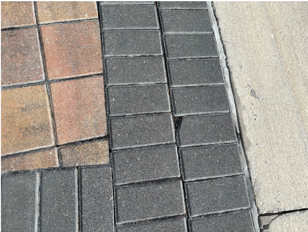
Photo 78 - Broken Concrete Pavers on Truck Apron
