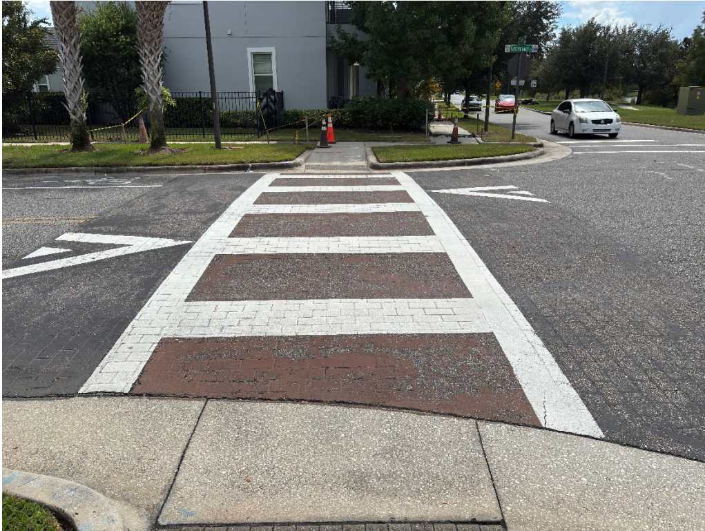
Photo 35 - Deteriorating Thermoplastic and Worn Crosswalk Coloration
