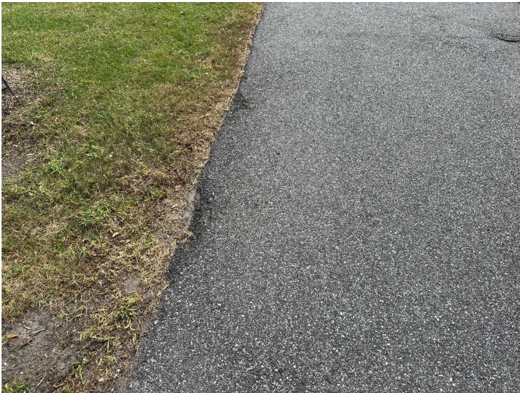
Photo 4 – Asphalt Pavement Edge Failure
