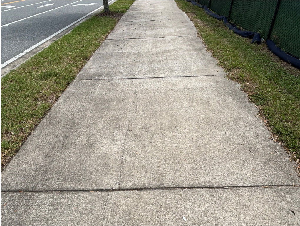
Photo 29 – Surficial Cracked Concrete
