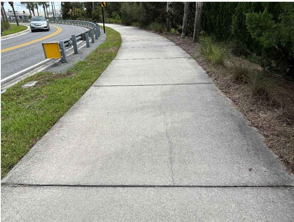
Photo 26 – Surficial Cracked Concrete
