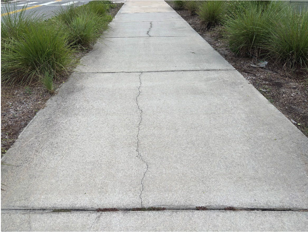
Photo 23 – Surficial Cracked Concrete
