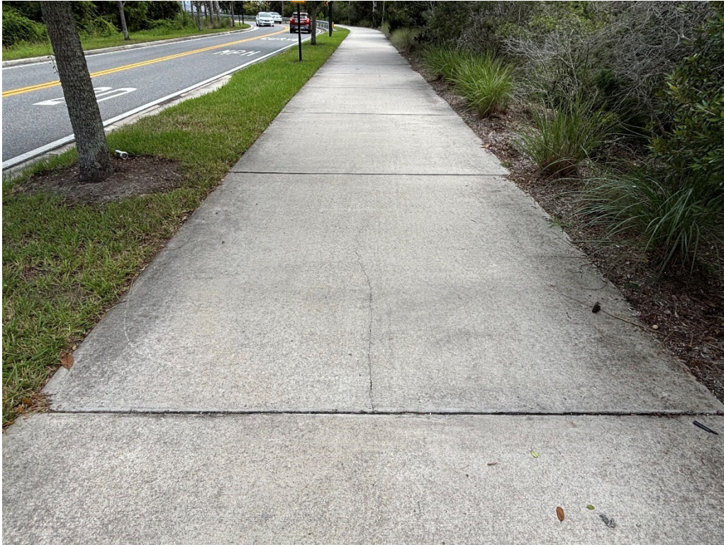
Photo 25 – Surficial Cracked Concrete
