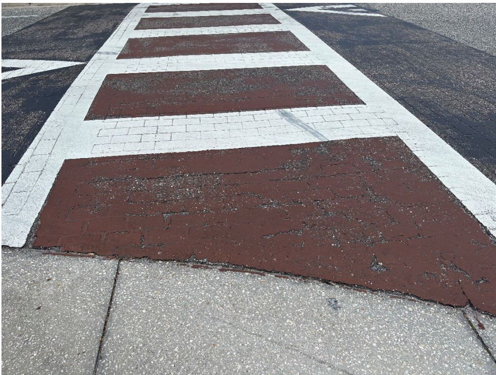
Photo 54 – Deteriorating Thermoplastic and Worn Crosswalk Coloration
