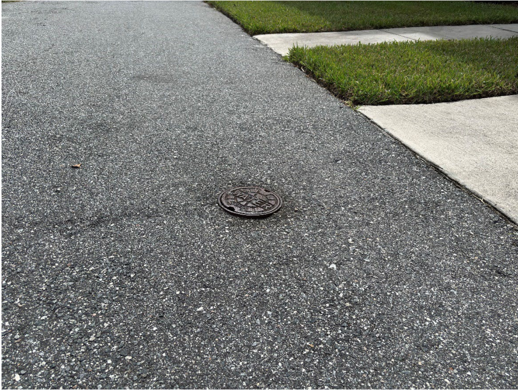
Photo 3 – Valve Cover Approximately 1 inch Reveal
