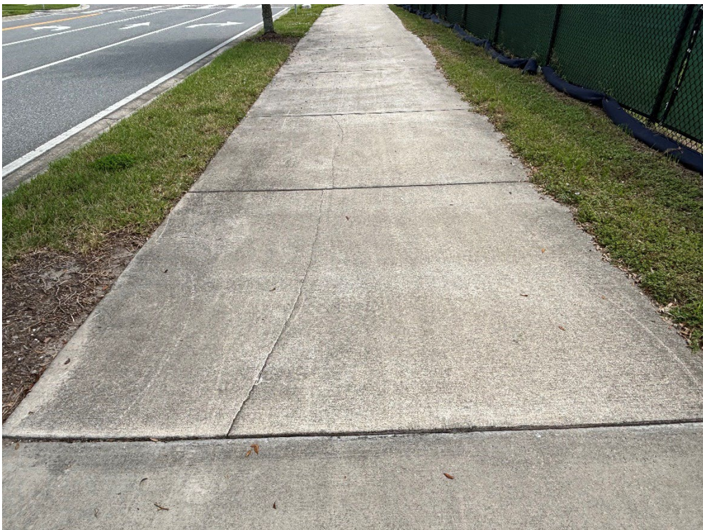
Photo 28 – Cracked Concrete
