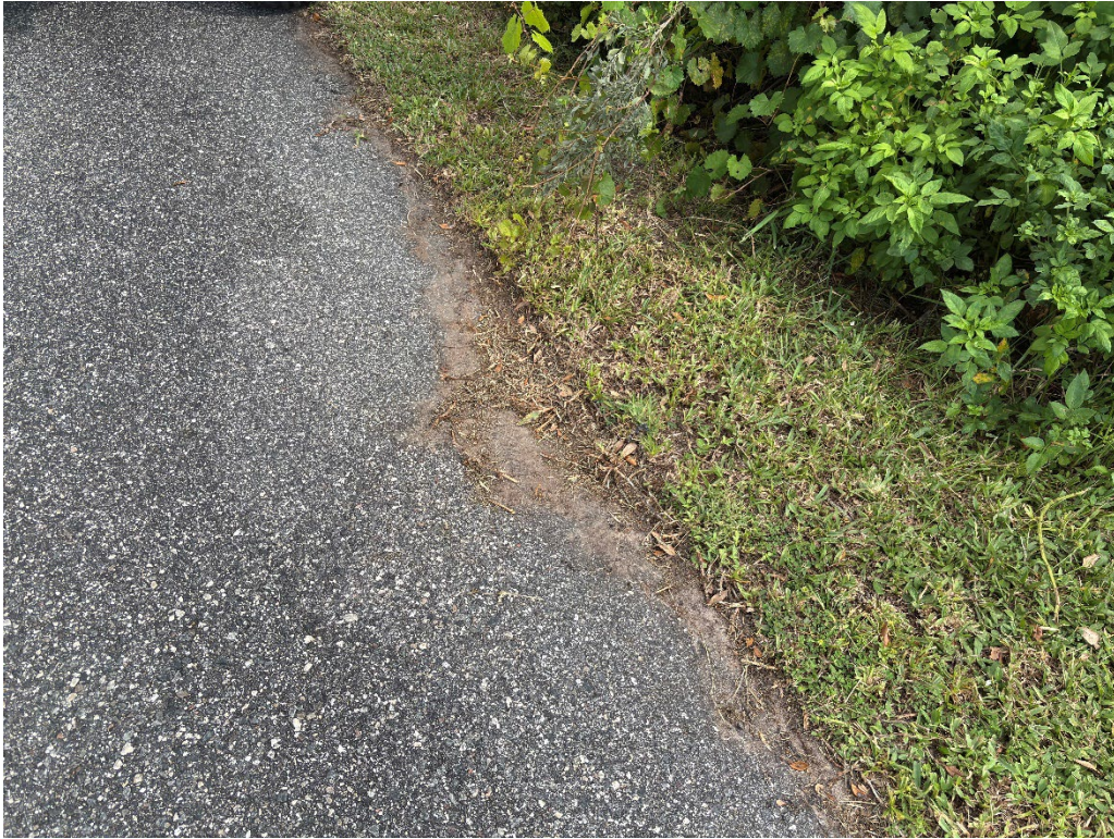
Photo 67 – Asphalt Edge Failure
