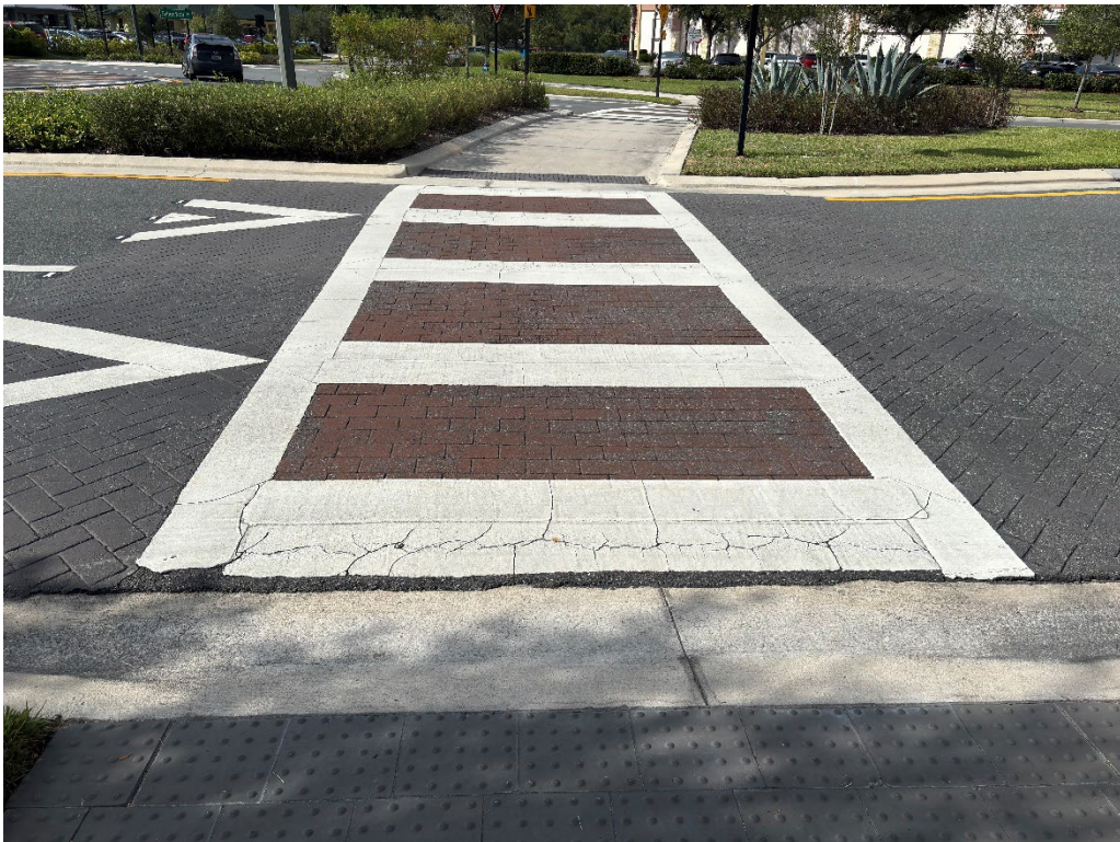
Photo 74 – Deteriorating Thermoplastic and Worn Crosswalk Coloration
