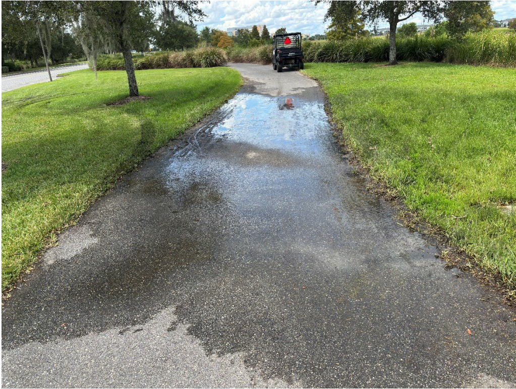
Photo 45 – Asphalt Raveling in Low Area
