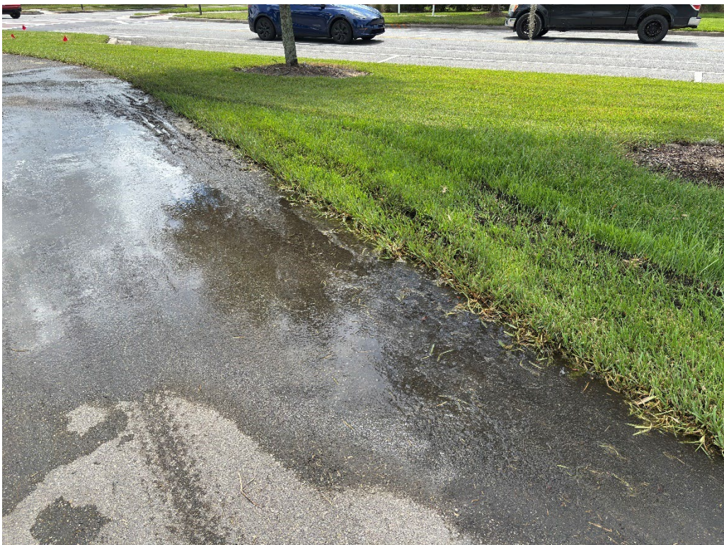
Photo 46 – Asphalt Raveling in Low Area
