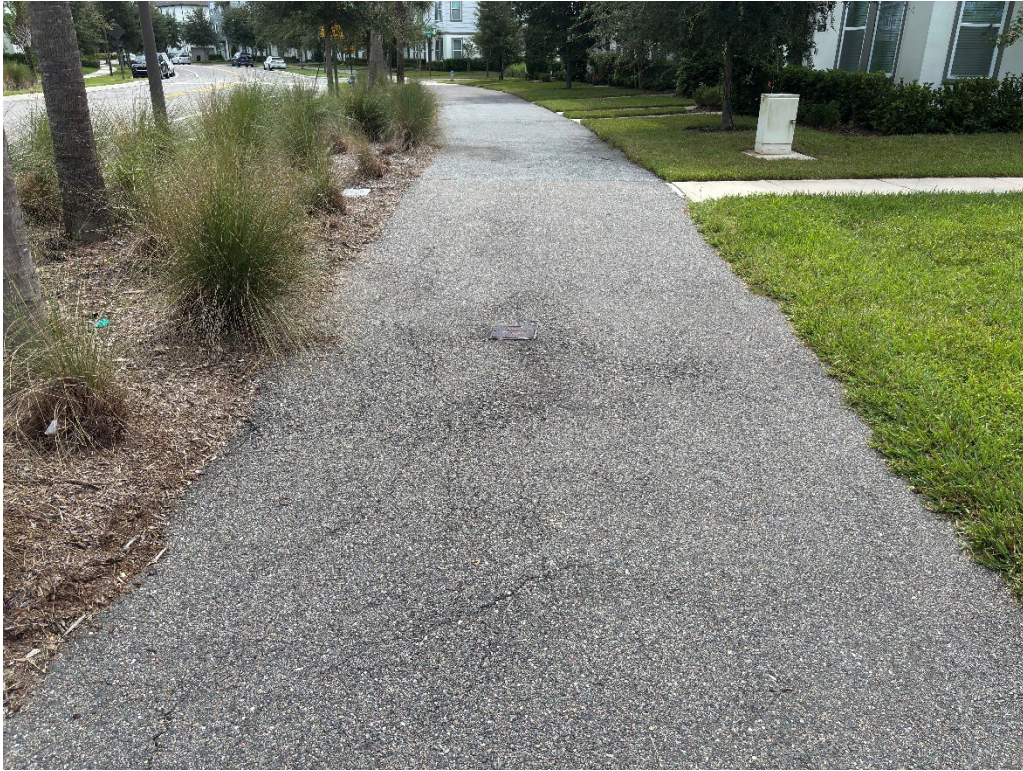
Photo 1 – Asphalt Raveling
