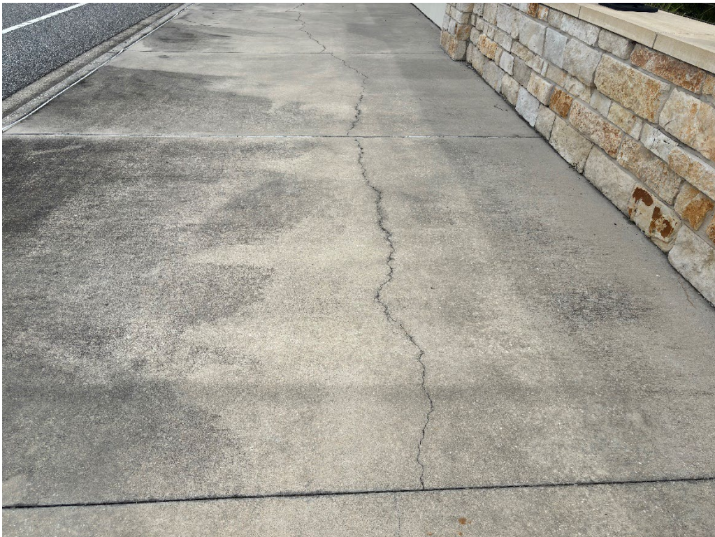
Photo 68 – Surficial Cracked Concrete
