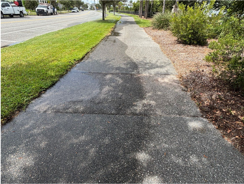
Photo 33 – Poor Quality Asphalt Patch
