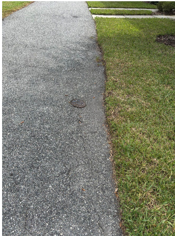
Photo 2 – Asphalt Pavement Edge Failure
