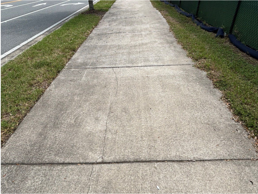
Photo 29 – Surficial Cracked Concrete
