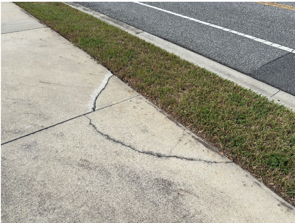
Photo 72 – Cracked Concrete and Base Failure
