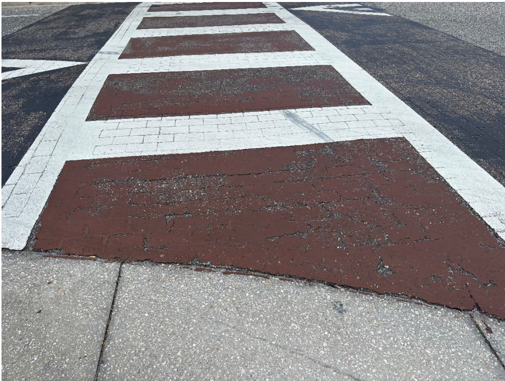
Photo 54 – Deteriorating Thermoplastic and Worn Crosswalk Coloration
