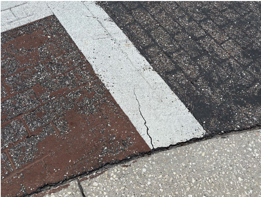
Photo 36 – Deteriorating Thermoplastic and Worn Crosswalk Coloration
