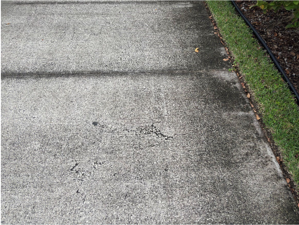
Photo 13 – Surficial Cracked Concrete
