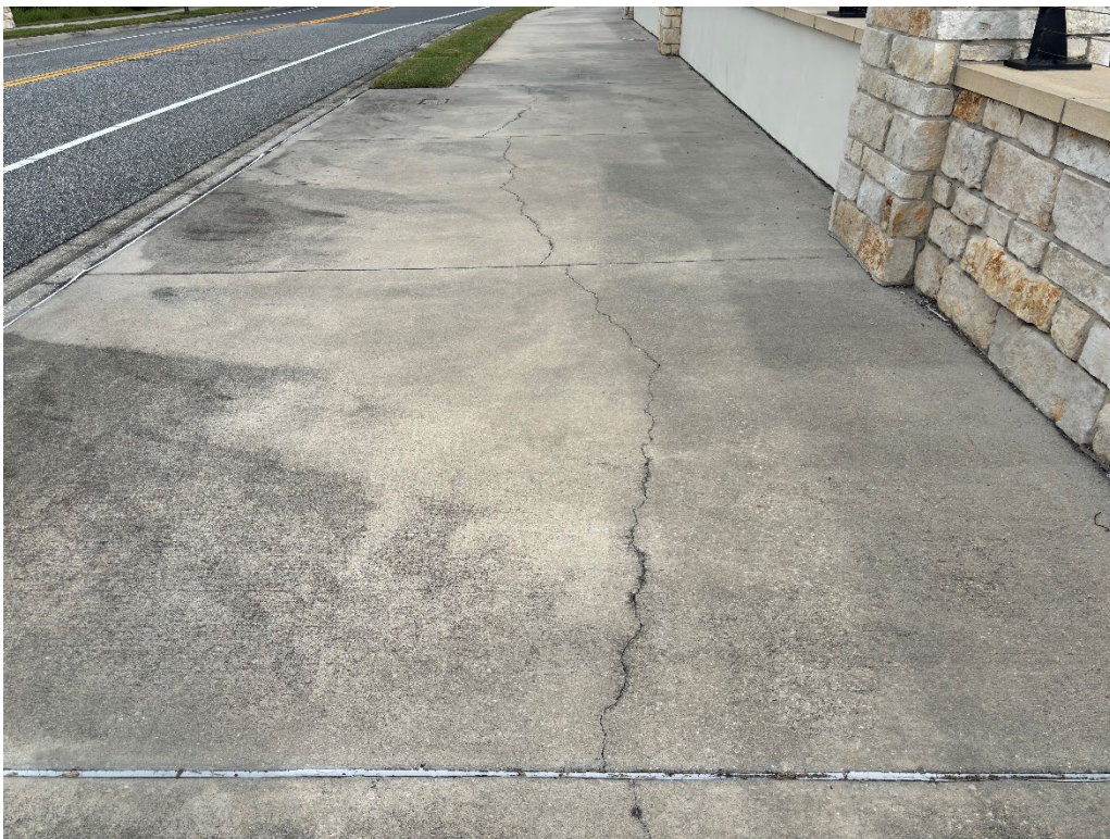
Photo 69 – Surficial Cracked Concrete
