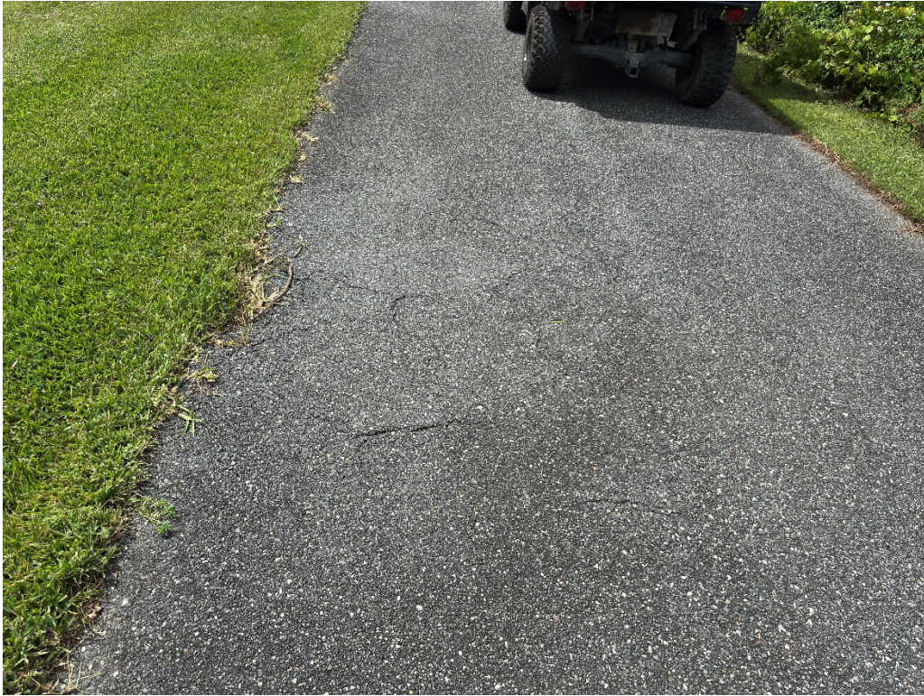
Photo 31 – Asphalt Raveling and Base Failure
