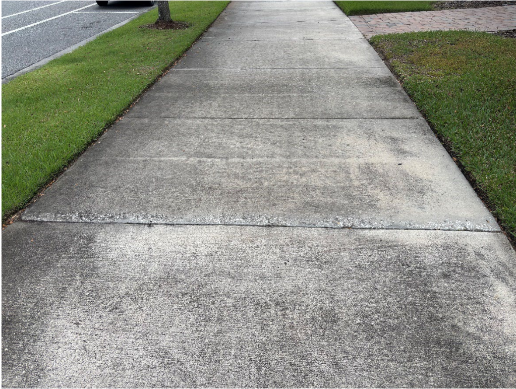
Photo 11 – Concrete Slab Movement (Previously Ground Down)
