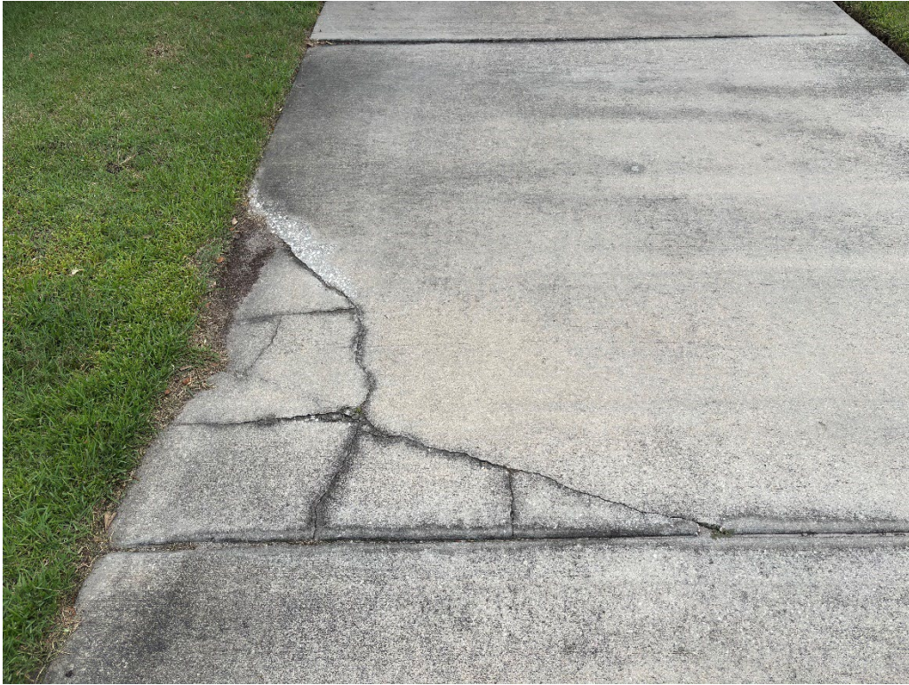
Photo 19 – Cracked Concrete and Base Failure
