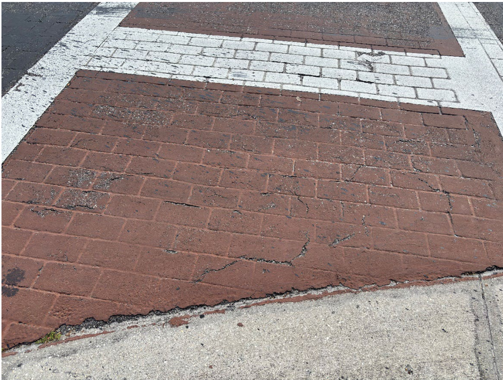
Photo 52 – Deteriorating Thermoplastic and Worn Crosswalk Coloration
