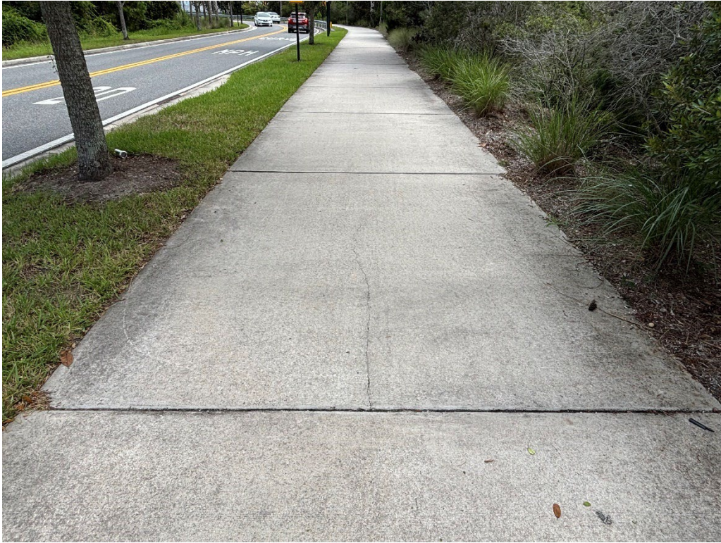
Photo 25 – Surficial Cracked Concrete
