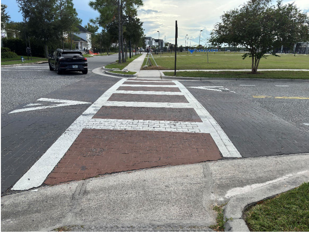
Photo 51 – Deteriorating Thermoplastic and Worn Crosswalk Coloration
