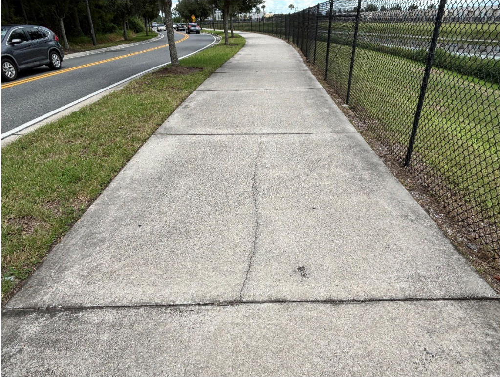
Photo 27 – Surficial Cracked Concrete
