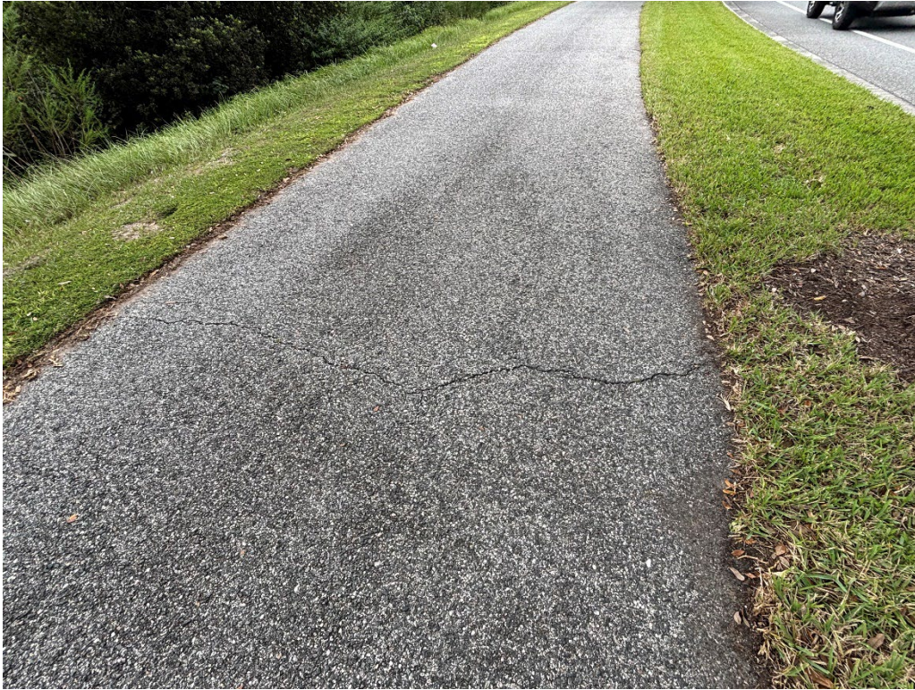
Photo 65 – Cracked Asphalt from Side to Side
