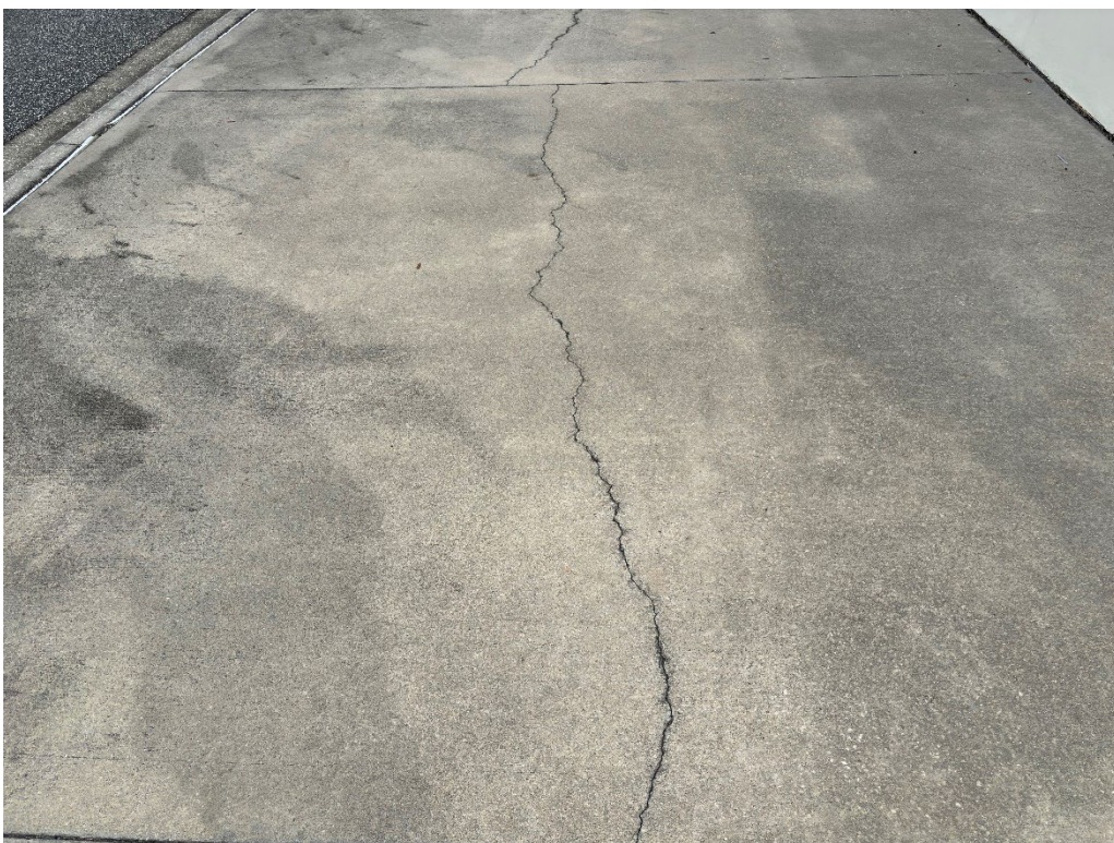
Photo 70 – Surficial Cracked Concrete
