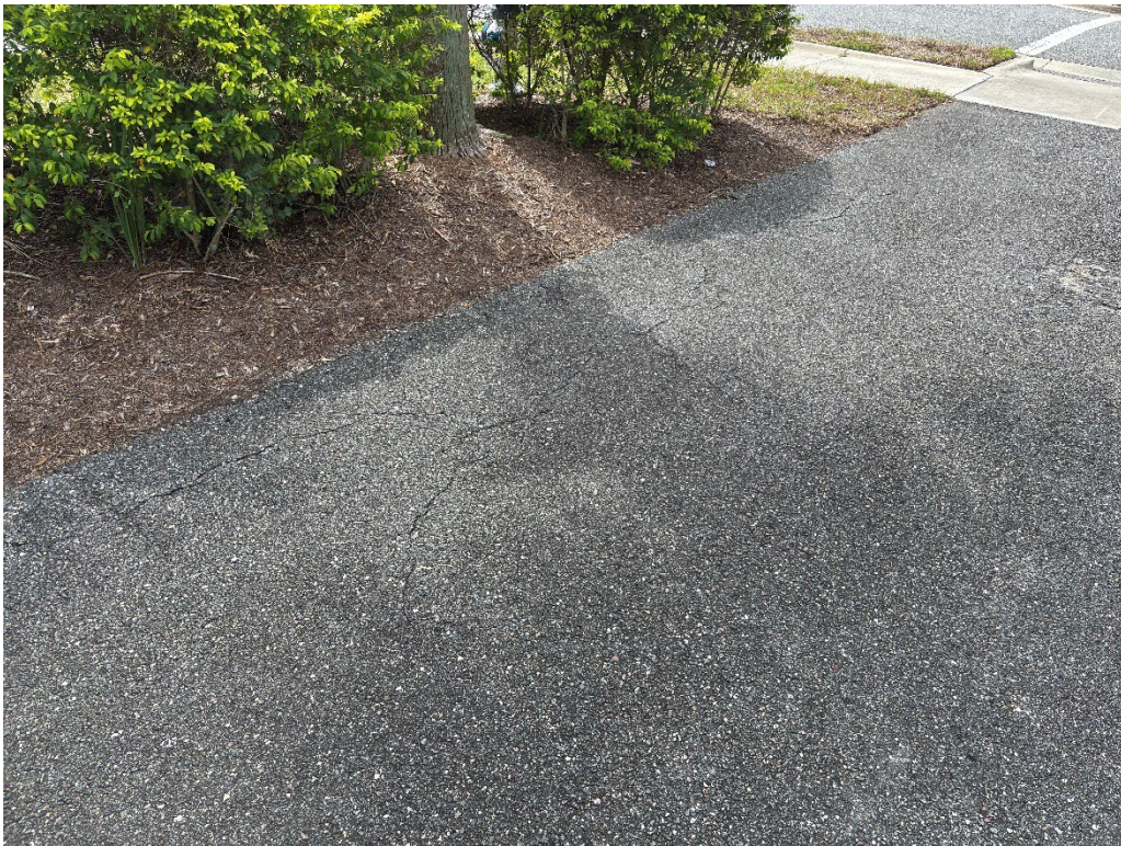
Photo 34 – Asphalt Raveling
