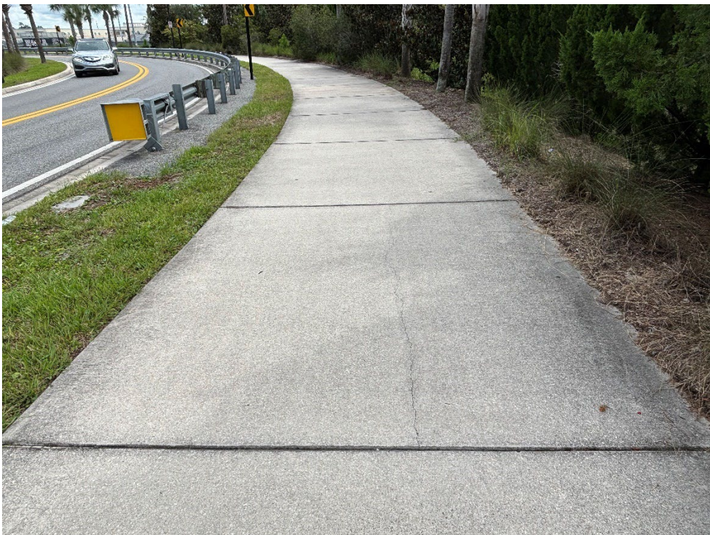
Photo 26 – Surficial Cracked Concrete
