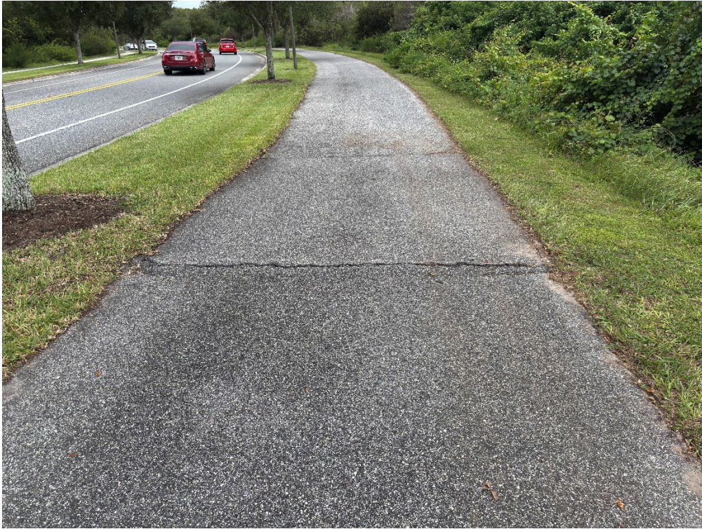
Photo 63 – Asphalt Patch Lifting
