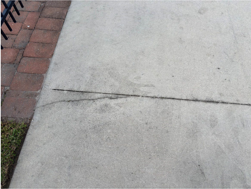
Photo 17 – Surficial Cracked Concrete
