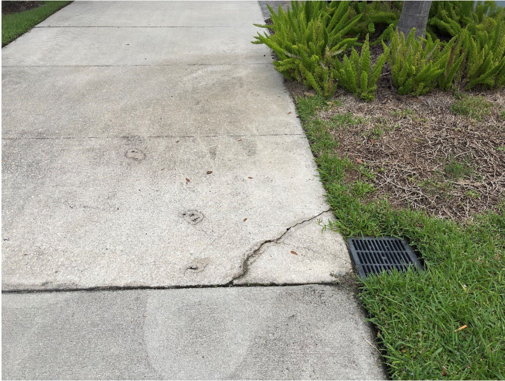
Photo 15 – Concrete Failure at Inlet
