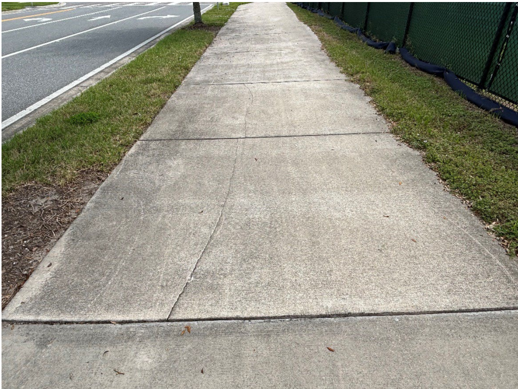
Photo 28 – Cracked Concrete
