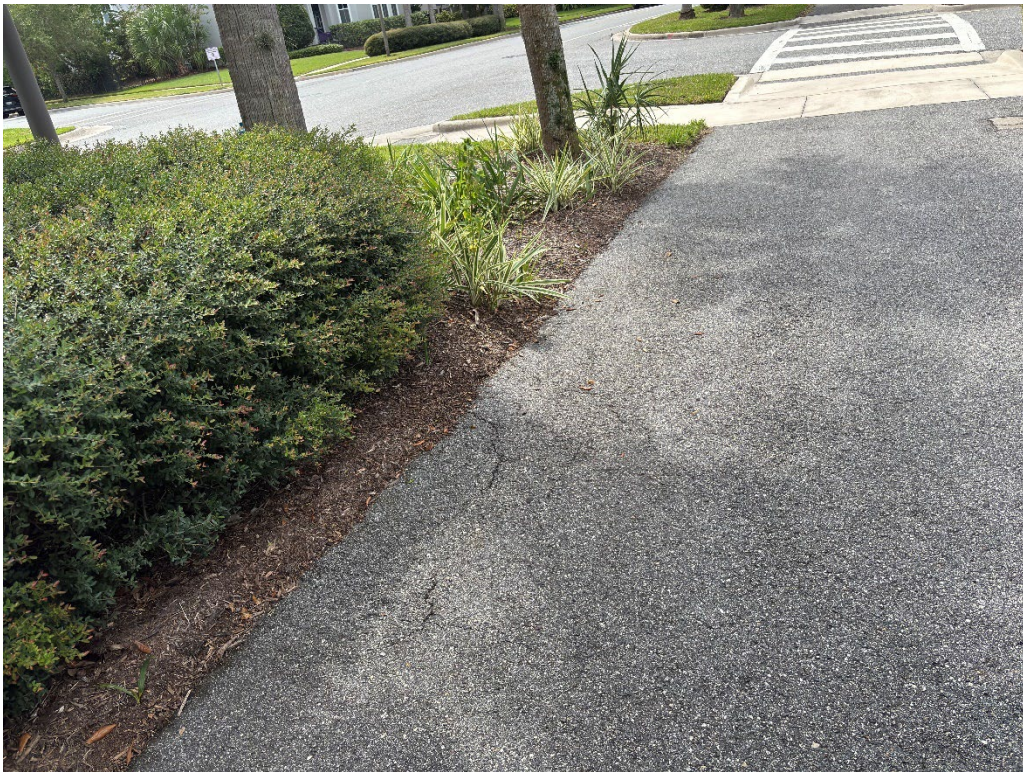
Photo 40 – Asphalt Raveling
