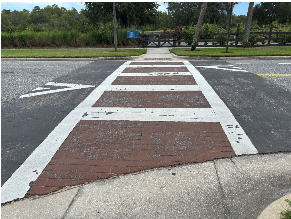
Photo 56 – Deteriorating Thermoplastic and Worn Crosswalk Coloration
