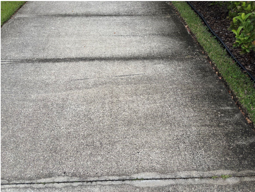
Photo 12 - Surficial Cracked Concrete
